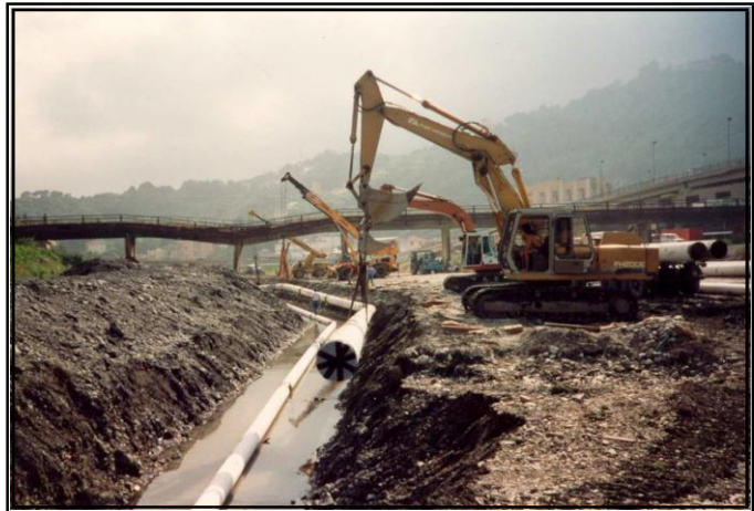
Oil Pipelines installation Polcevera Genova
