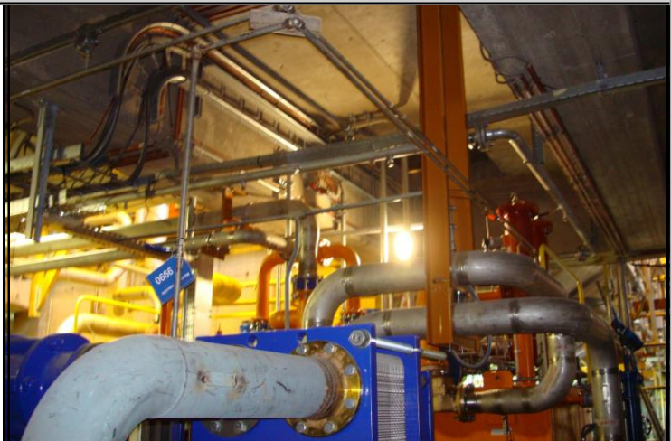
Pressure Parts Installation - Amercoeur Power Plant
